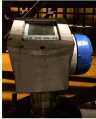
Gambar 4. Level Transmitter
